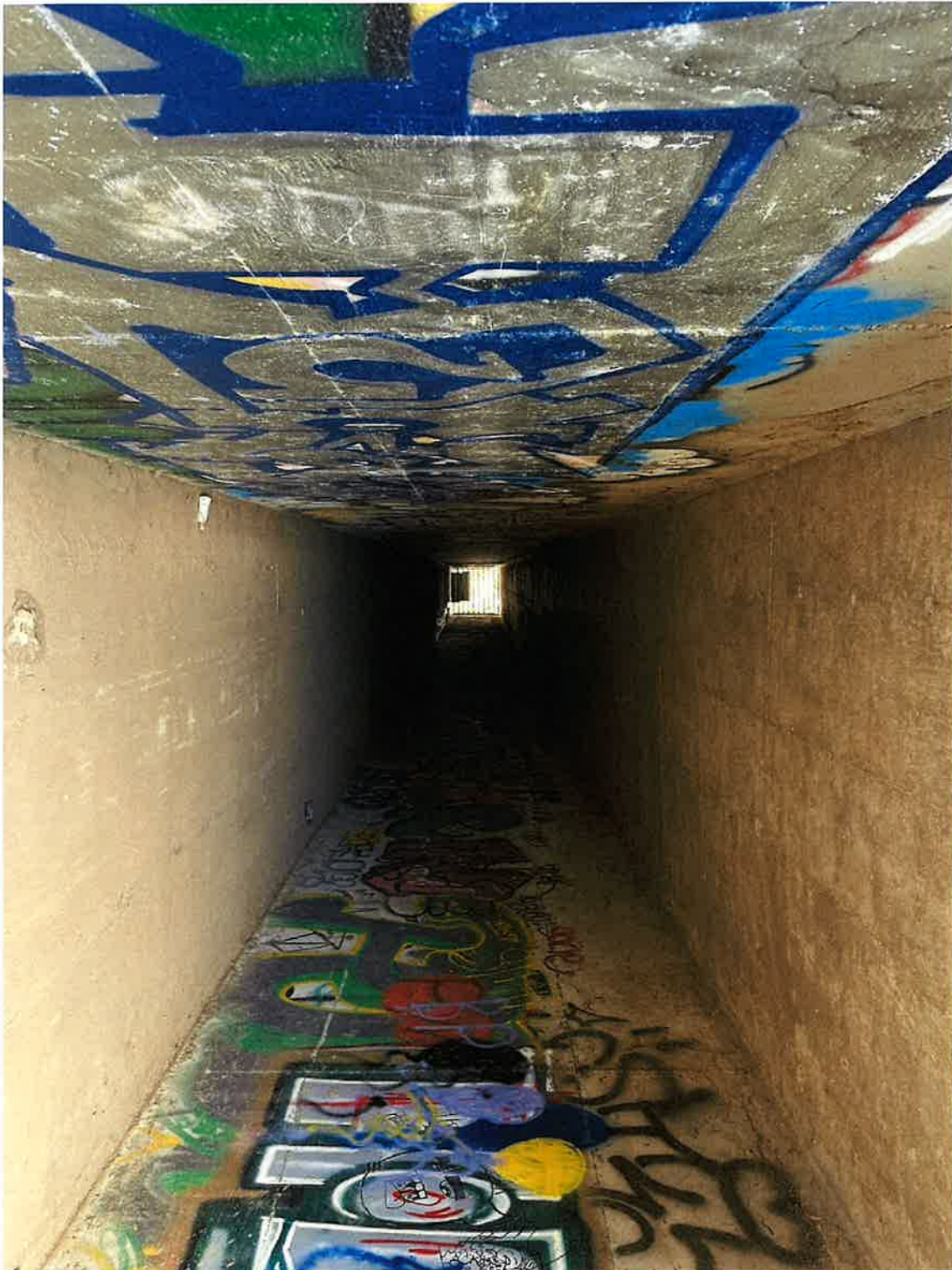
No signs of intrusion since the installation of the Eco blocks at both ends of the tunnel, near Sta 770+50.
