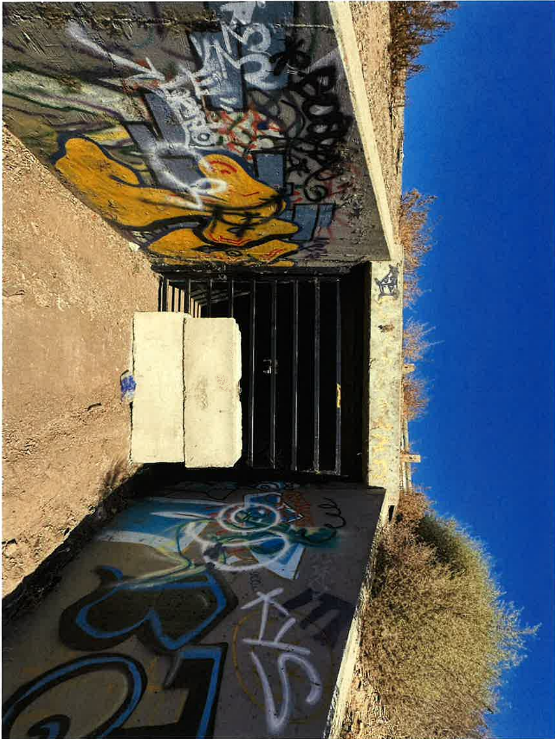
EcoBlocks at the south end of the tunnel at Sta 770+50 - No signs of intrusion or intrusion attempts since the installation of the blocks.
