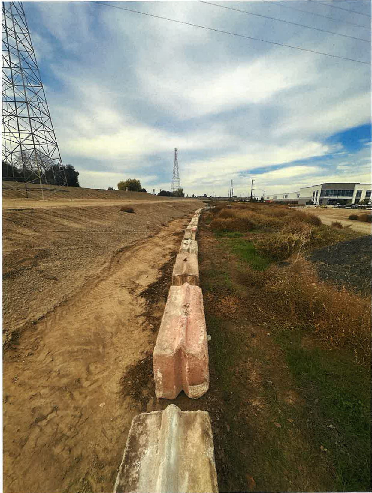
Figure 9. 0856-9026 - EW Black placed (96) ecoblocks along levee toe to prevent unauthorized access to the levee near Sta 795+00.
